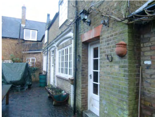
Picture 1.27 Original recessed doorway with gauged brick arch above - mirrored on the other side
