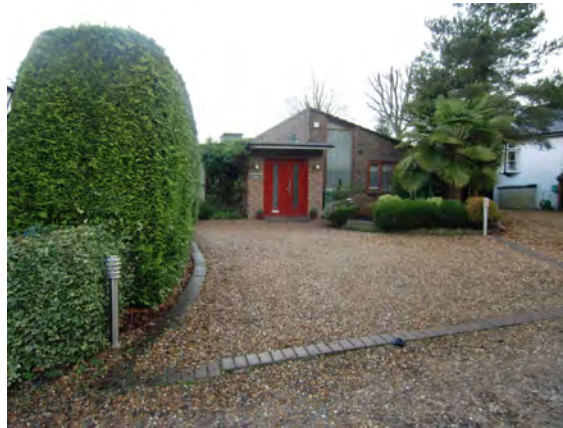
Picture 1.49 44a West Drive
