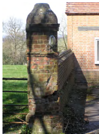
Picture 1.48 Curtilage listed entrance pier to the stable block
