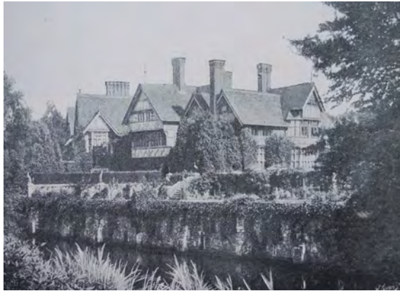
Picture 1.11 Grim's Dyke Hotel 1891
