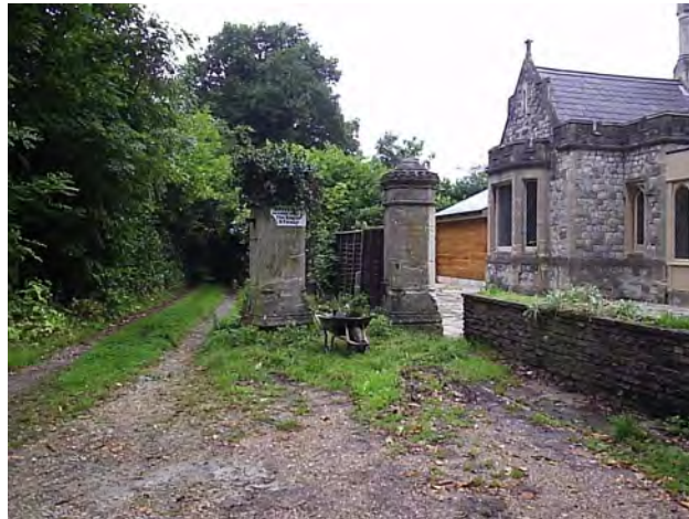
Picture 1.32 Two of the listed gate piers and the locally listed North Lodge
