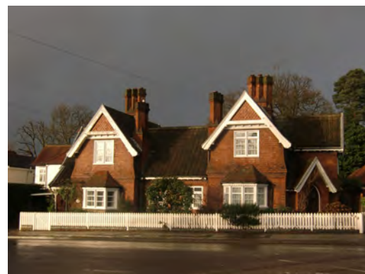
Picture 1.48 148 and 150 Uxbridge Road (former Gamekeeper's lodge)
