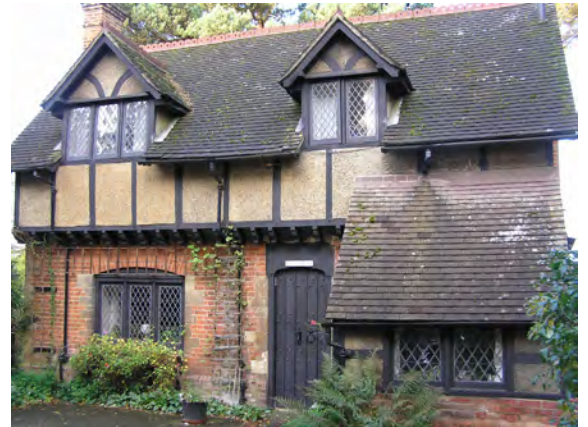
Picture 1.39 North Lodge LBH LA.100019206.2013
