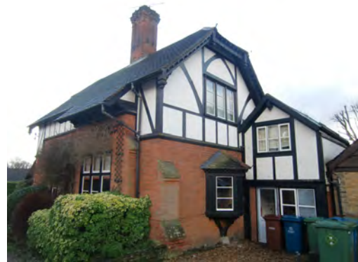
Picture 1.35 View looking south towards 47 West Drive
