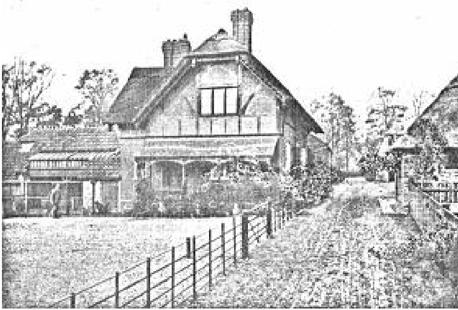
Picture 1.33 19th century photograph of the farm house
