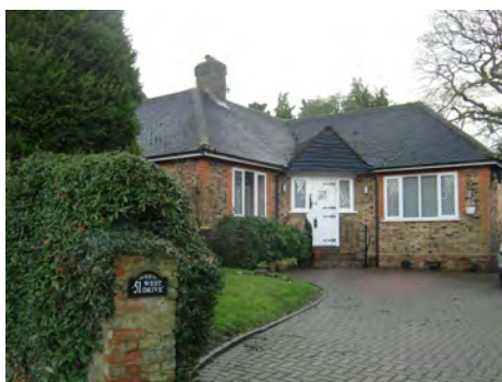
Picture 1.50 51 West Drive
