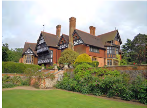
Picture 1.12 Grim's Dyke Hotel 2013
